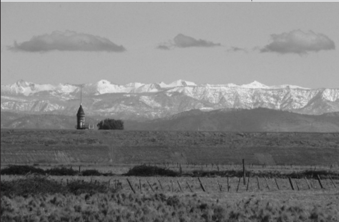
The Sierra Nevada provides a majestic backdrop for the water tower at Lake Yosemite.
