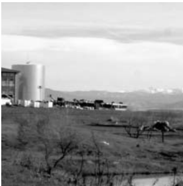
Little Lake, with the TES tank in background, key to campus energy savings.
